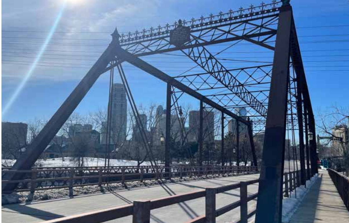
MERRIAM STREET BRIDGE
