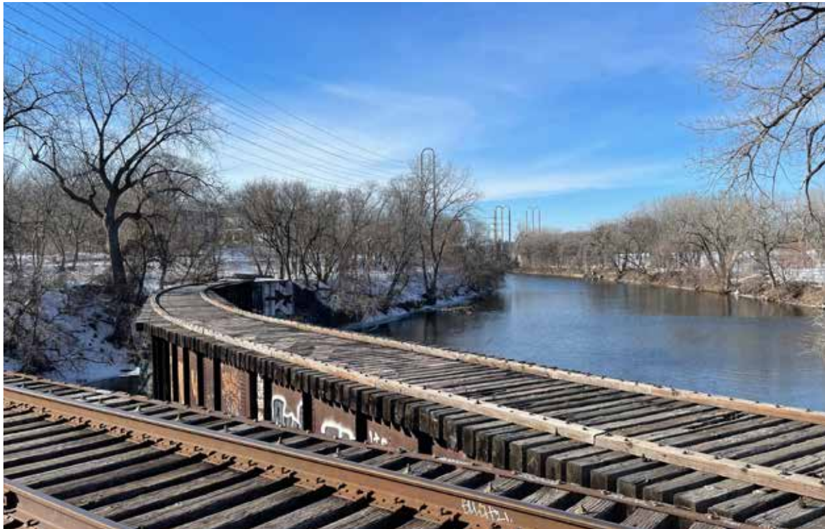
NICOLLET ISLAND RAILROAD BRIDGE
